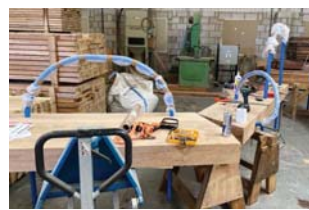
Off-site fabrication Spring 2020
