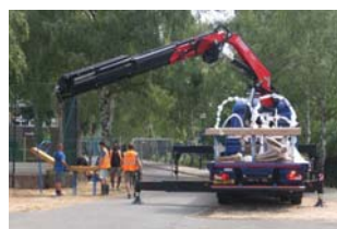
Site installation Summer 2020
